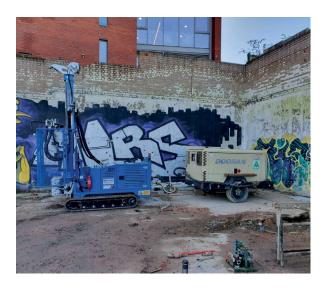
the ordnance. Eventually, the nose slows sufficiently that a bomb can level out – but it can also mean that the bomb actually comes back up again in a J shaped curve, driven by the tail. Bombs can travel underground for between 5 and 10m meaning they can come to rest underneath otherwise unaffected buildings. When we survey using a rig like the MI3 we always include a buffer zone in addition to the risk zone to cover off on the J curve effect.
